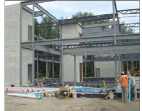
Construction continues on the new Providence Field Office located in Johnstown, RI. Interior stairwells have been laid up, structural steel is being erected and site work continues. Anticipated occupancy is in December 2008.
